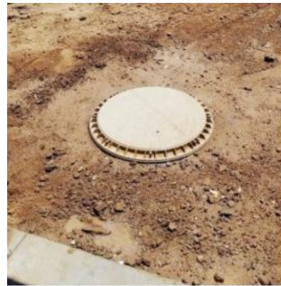
Riser Lid - Proper Pumping Port
